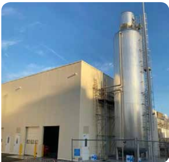
Hot water grid - 85% complete
