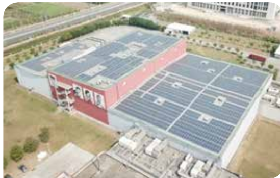
China 912kWp of solar panel = 6000m 2
