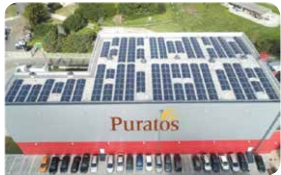
Portugal 130kWp of solar panel = 800m 2
